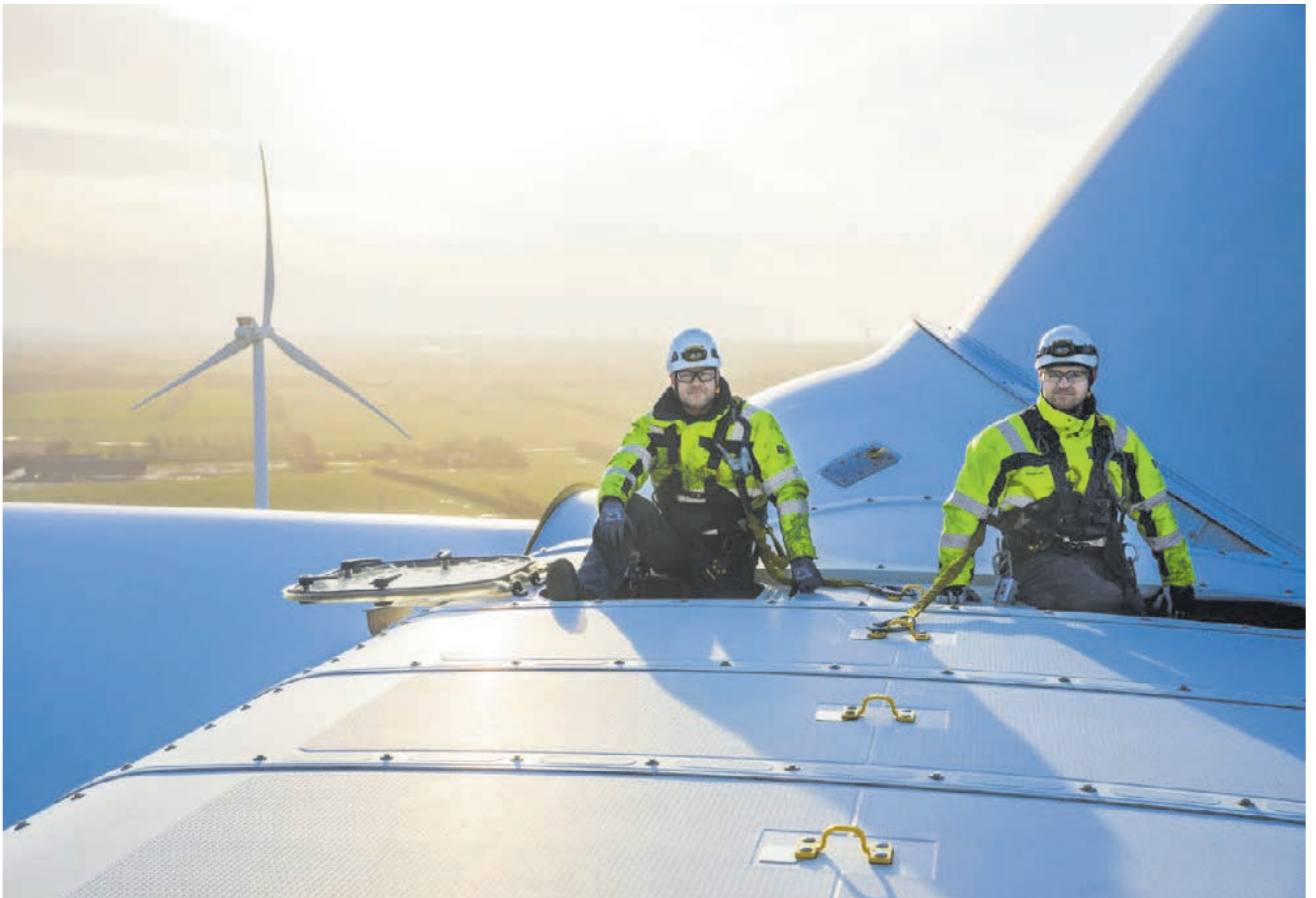
Photo Courtesy of Vestas Wind Systems A/S
